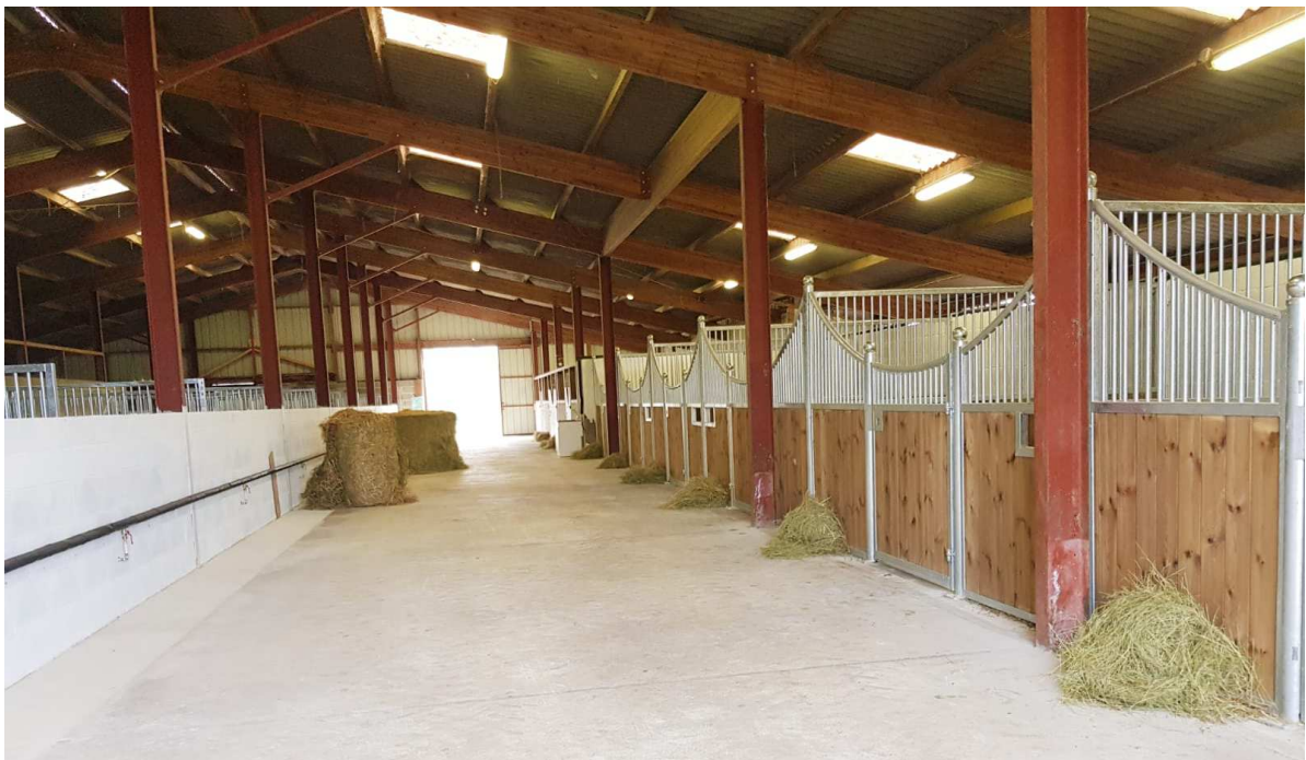
Photo: Former Limousin cattle barn has been reconstructed into a well-areated horse barn with 26 large boxes.
