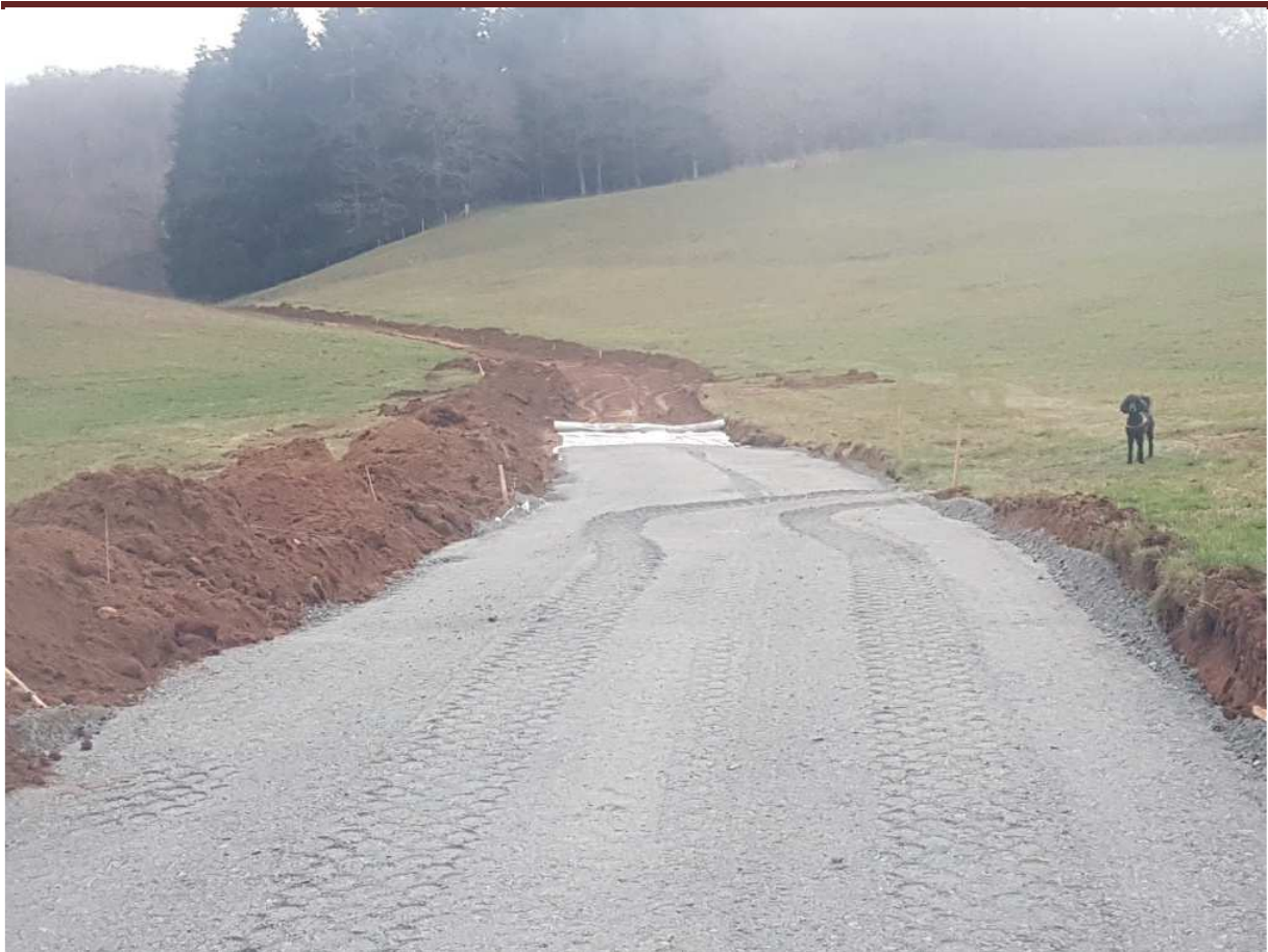
Photo: Uphill training track under construction: 1200m, uphill on last 600m.
