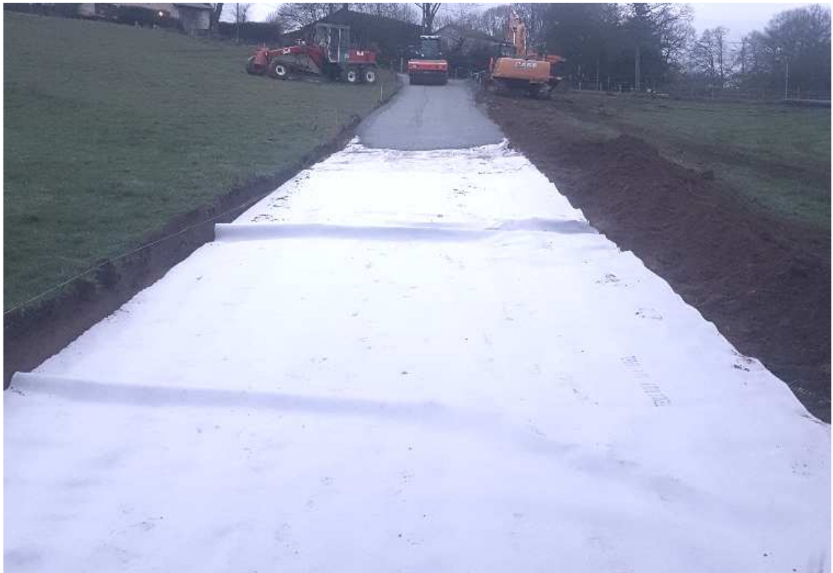
Photo: Geotextile surface and gravel as base for the wood chips.
